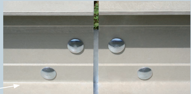
Mushroom-head bolts, maintained expansion gap
