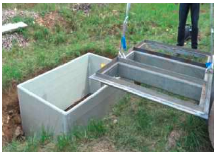
4. Place the cover frame on the cable junction box using a suitable lifting gear.
