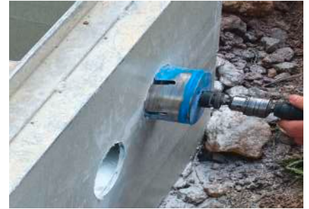
3. Use a hole saw to drill the wall for the connections of the pipes. Do not drill through the lower ring.
