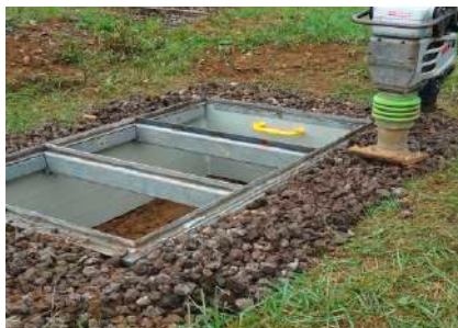
5. Fill the excavation flush up to the frame and compact with a vibratory tamper.
