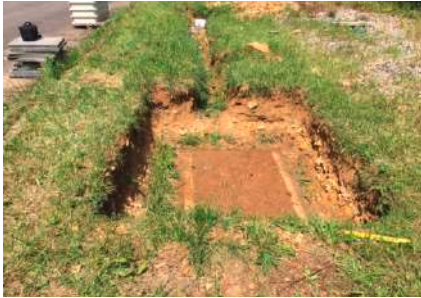
1. Preparation of a stable and even subfloor.
